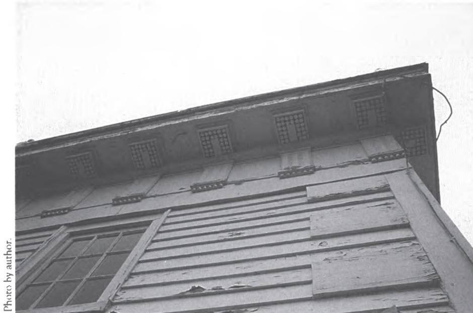
8-7. Detail of tower, Kirtland Temple, ca. 1992. Originally, the triglyphs of the Doric entablature would have been backed up by thick planking. The planking was replaced with thin composition board, which visibly bows over the window. Also note the overlapping clapboard, which replaced the original flushboard siding.
