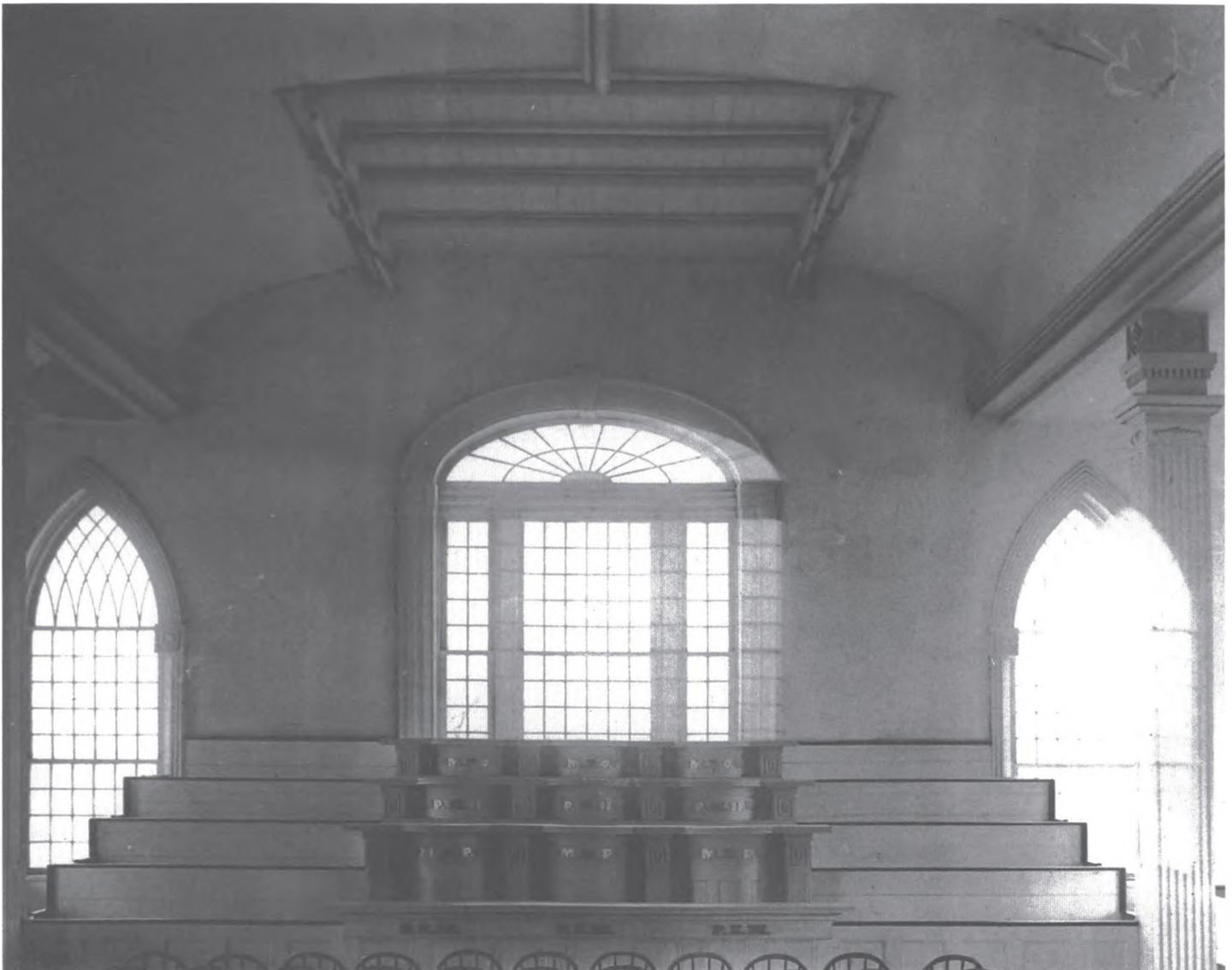
**8-10.** Upper court looking west, photograph by George Edward Anderson, August 1907. Cracking at the junction between the ceiling and the west wall mirrors that shown in Fig. 6-1 although the cracking is not as extensive. Also note the missing plaster in the ceiling to the left. Chairs were used in the upper court before pew boxes imitating those in the lower court were installed sometime between 1918 and 1931.
