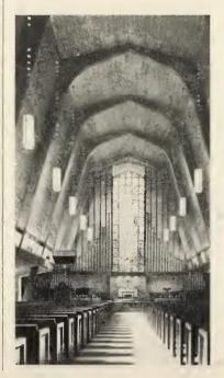
Rilco laminated wood arches and beams are a natural for a house of worship. The warm hues and subtle grain patterns create a dramatic architectural character unduplicated by any other material. Initial cost is low, erection is fast and maintenance costs minimal. To give you interesting ideas on the use of laminated wood, a Rilco Church Construction booklet also accompanies the Church Architect booklet.
